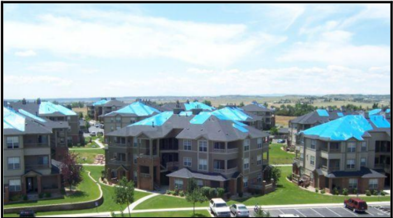
Figure 1 Photo shows example of extensive tarping applied to damaged roofs throughout complex. A total of 29 buildings were covered by the authorized emergency tarping efforts performed by Weather Guard Construction Company (WCC).
